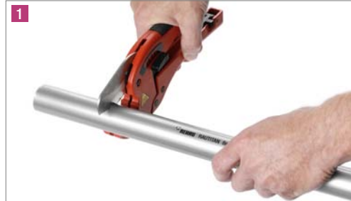
1. Cut the pipe
